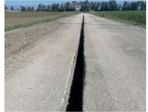
Scavo in minitrincea
